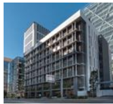
(TO-16) A-PLACE Shinagawa Higashi
