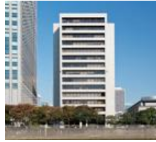
(AA-7) Osaka Nakanoshima Building
