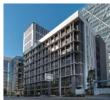
(TO-16) A-PLACE Shinagawa Higashi
