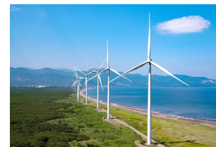
Wind energy plant in Hokkaido
