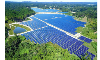
Photovoltaic power plant in Chiba
