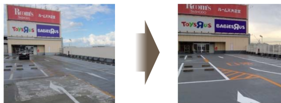
icot Mizonokuchi Renovation of water-resistant paint on the rooftop
