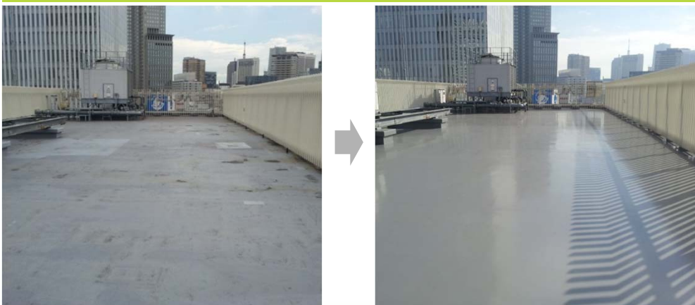
Tokyu Plaza Akasaka Renovation of water-resistant paint on the rooftop
