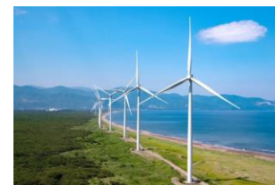
Wind energy plant in Hokkaido
