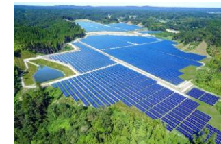
Photovoltaic power plant in Chiba
